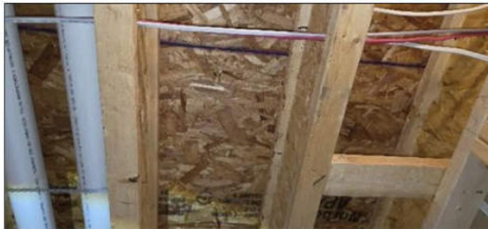
19. Subfloor - OSB (Oriented Strand Board)
